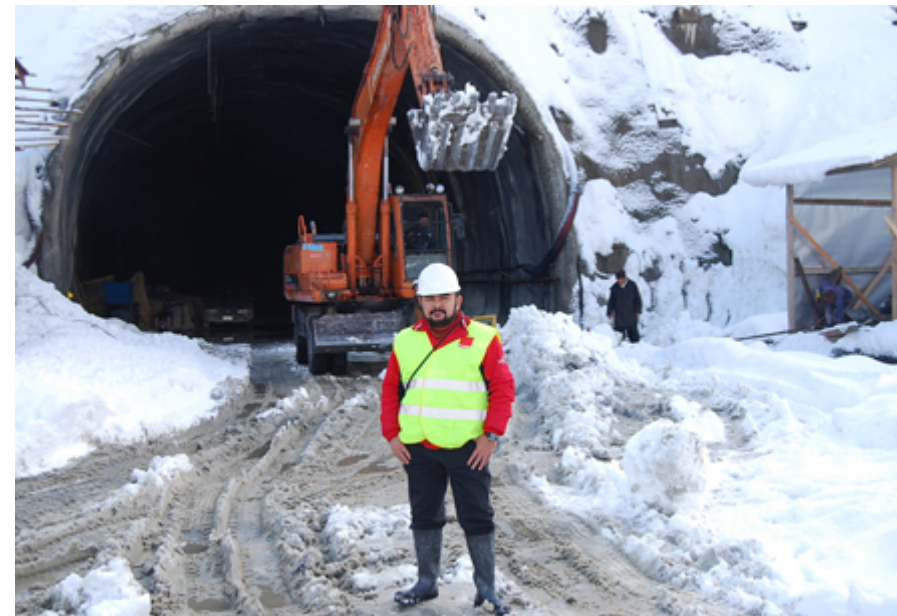
Glenn Amador Bautista, at north portal
