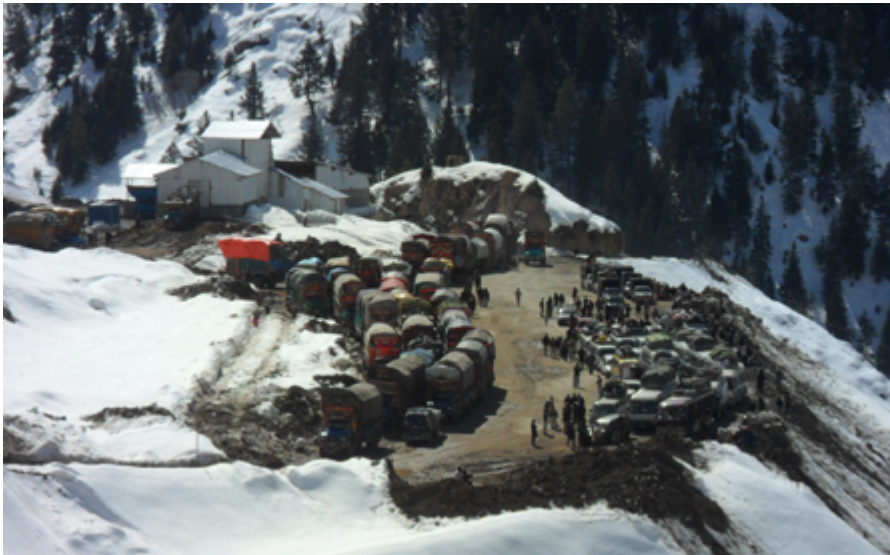
Vehicles at south portal, waiting to pass the tunnel
