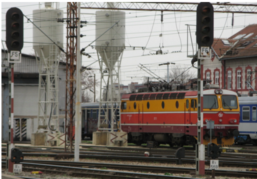
Zagreb Main Station: F-5, F-6 signals
