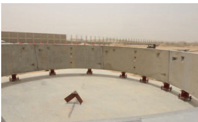
Tunnel lining segments in factory and tunnel lining assembly test
