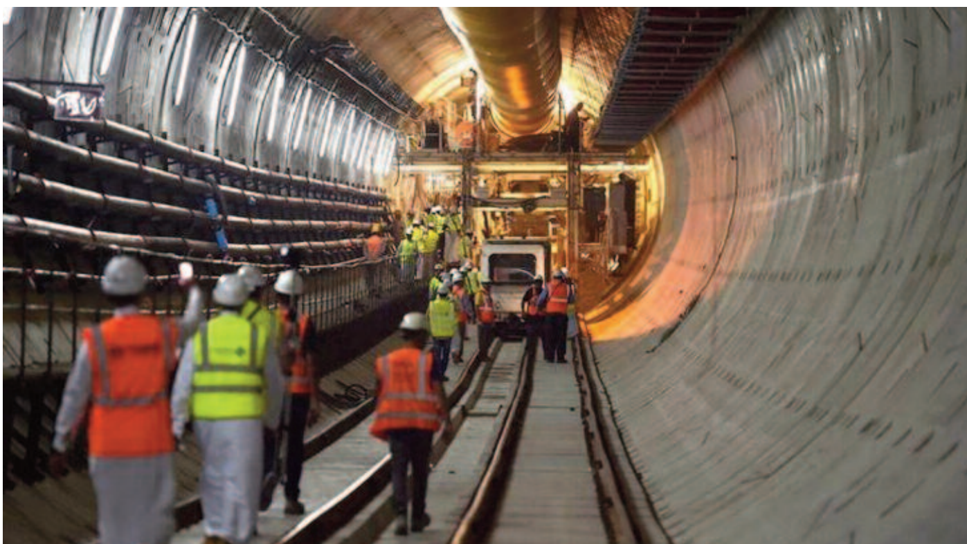
General overview of the tunnel and the assembled concrete rings
