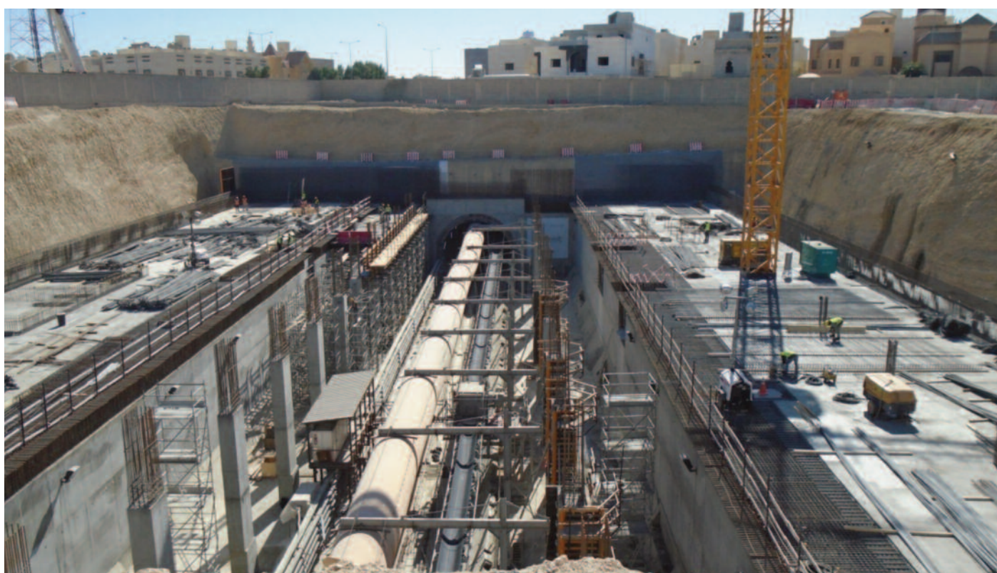
Structure, progressing in lateral span cast at site
