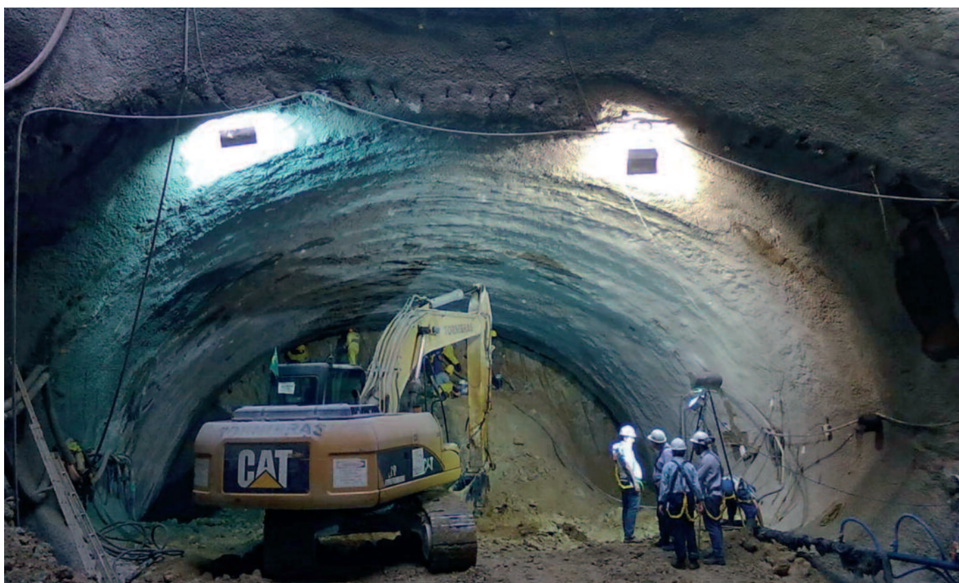
Portal of a tunnel weathered rock
