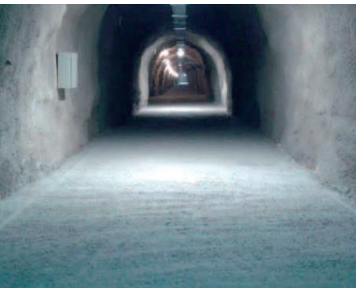
Emergency gallery and emergency exit
