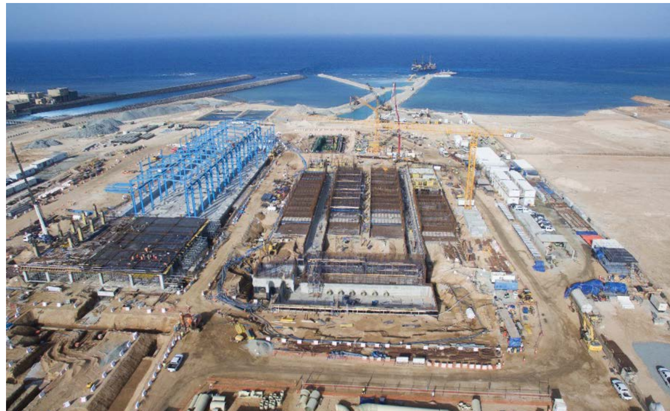
Aerial view Shuaibah 3 Expansion II SWRO, June 2018
