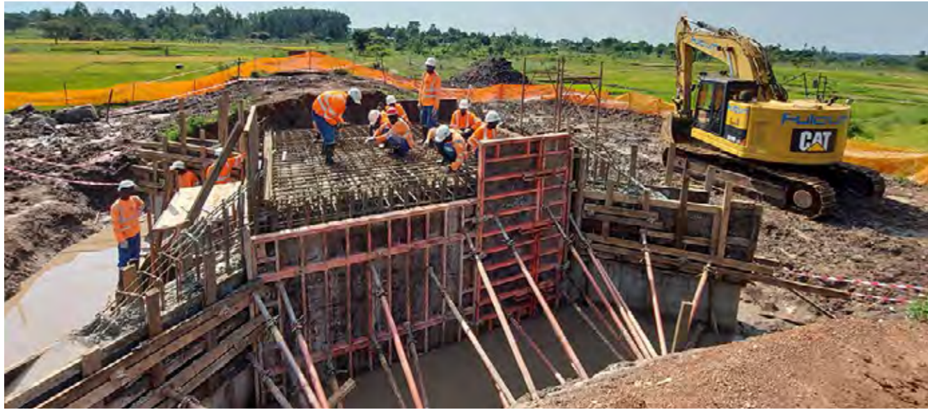
Construction of box culvert
