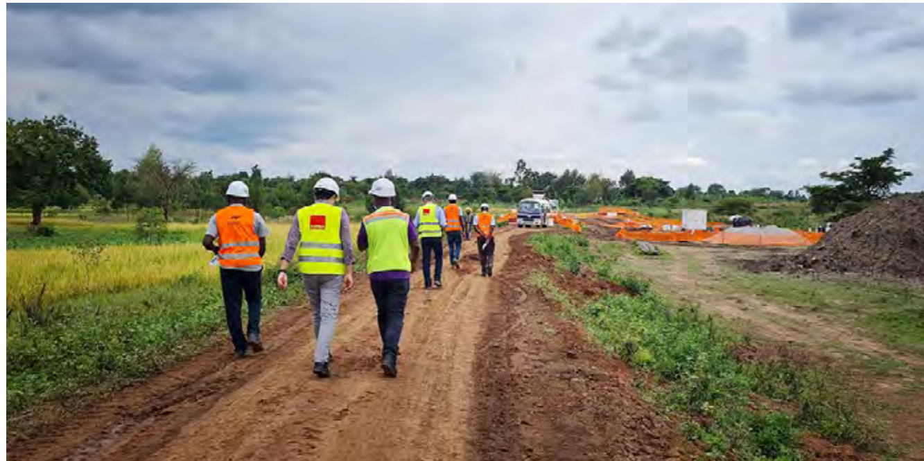
Site meeting / inspection
