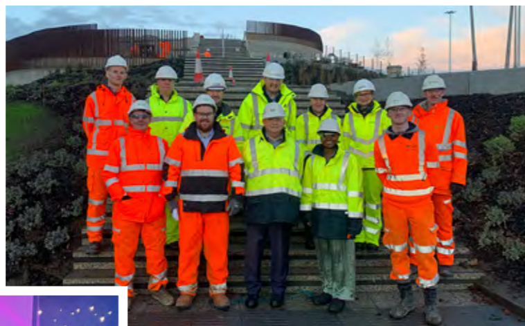
Site visit to footbridge over the M8 Motorway
