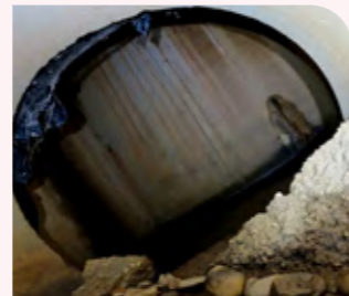
Culverts with large obstructions and rough terrain
