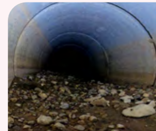
Culverts with large obstructions and rough terrain
