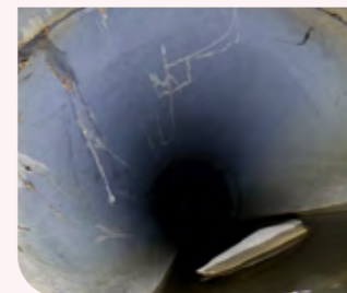
Partially submerged culverts with large obstructions
