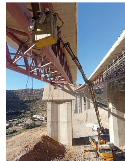
Reinforcement works on the Caballar viaduct. Almería, Spain
