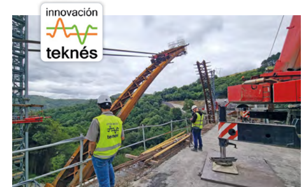
Monitoring the settlement of the Bolintxu viaduct
