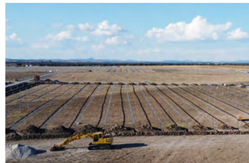
Implementation works at the Carmonita Sur solar photovoltaic park, Badajoz
