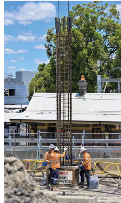
Metro works in Toronto, Canada
