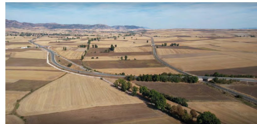
Intersection of the Piñerías-Pancorbo high-speed railway line with the N-1, Spain
