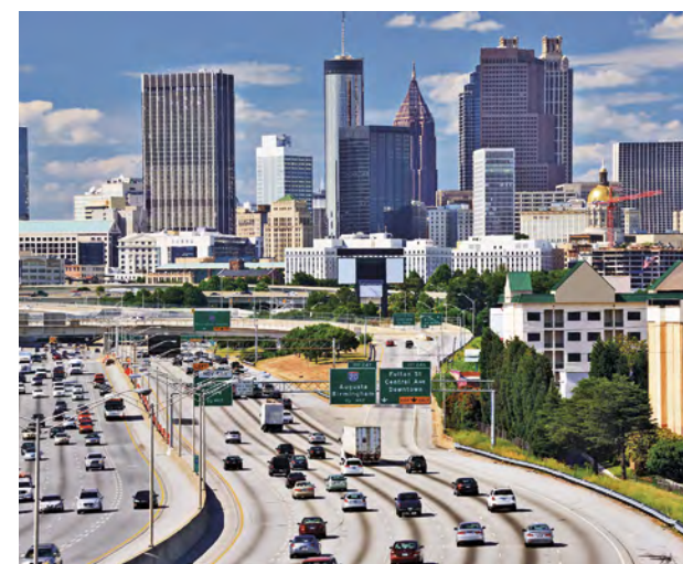
SR 400 Highway in Atlanta, Georgia
