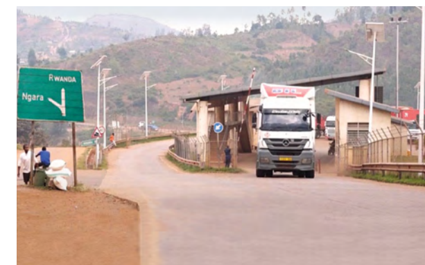
Rehabilitation of the road from Lusahunga to Rusumo in Tanzania
