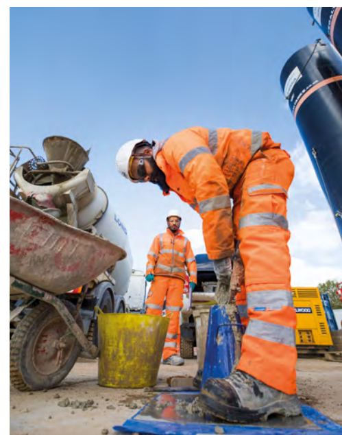
Works for HS2 High-speed railway in the United Kingdom
