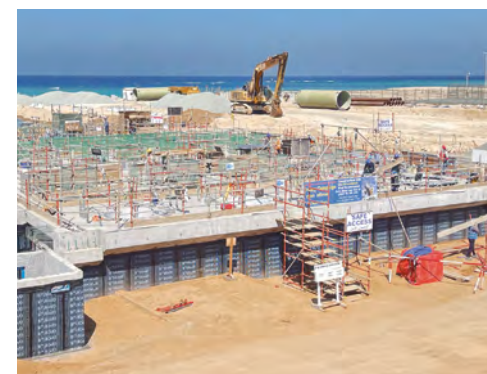
Works at the Shuaibah3 desalination plant, Saudi Arabia
