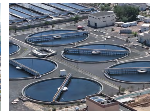
Madinah-3 wastewater treatment plant, Saudi Arabia
