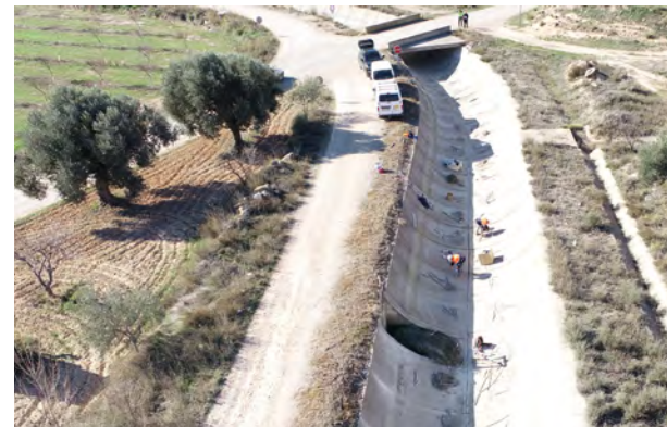
Conservation and maintenance of the Calanda-Alcañiz canal, Zaragoza,
