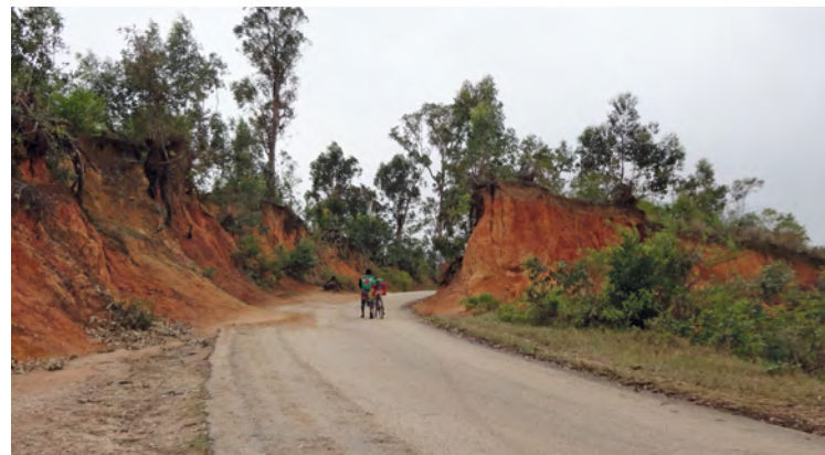
Road rehabilitation in Madagascar
