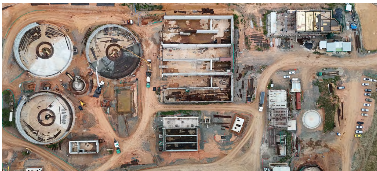
Construction of the wastewater treatment plant in Arraiján Este, Panama
