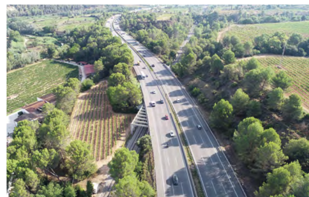
Widening of the AP -7 motorway, Barcelona
