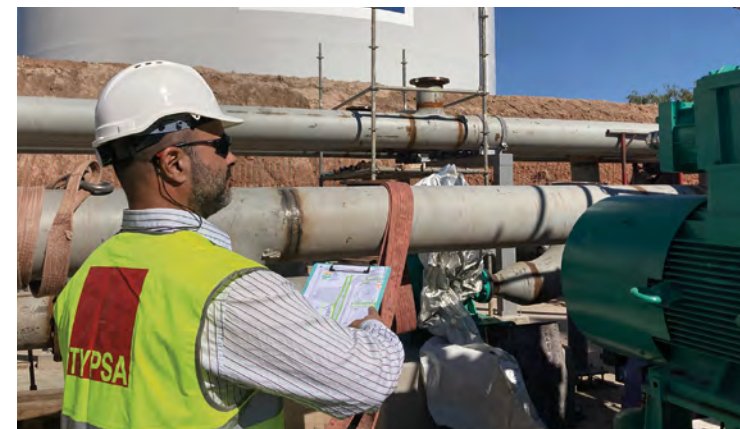
Extension of Nueva Palmira port bulk terminal, Uruguay
