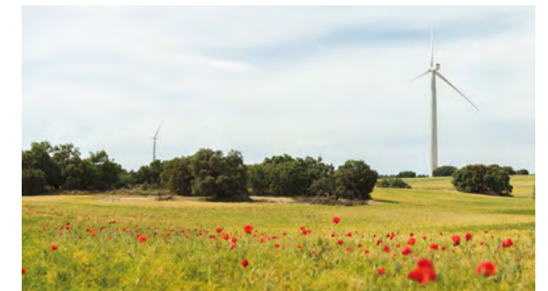
Gecama wind farm, Cuenca, Spain
