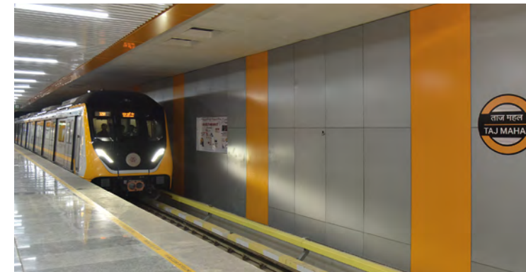
First section of the Agra metro network, India
