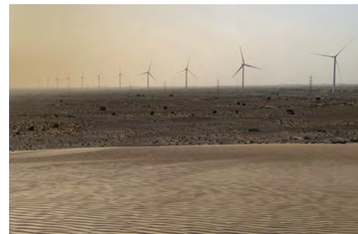
Wind farm in Boulouvar, Mauritania
