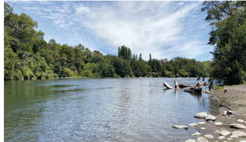
Las Vertientes-Púa irrigation system in the Araucania region, Chile
